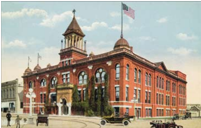
This 17,500 sq.ft. temple built in Fargo, North Dakota in 1902 featured a two-story auditorium with balcony capped by a 40 ft. diameter dome.
